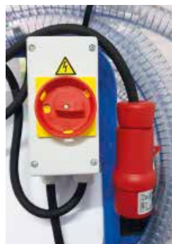
3-phase electrical panel
