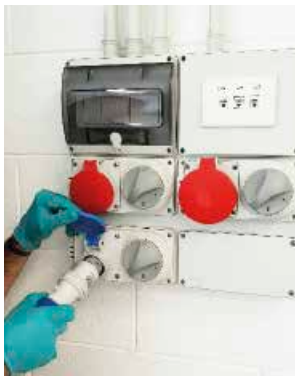
Electrical connection for the single-phase motor
