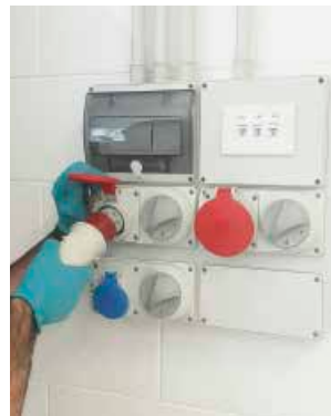
Electrical connection for the three-phase motor
