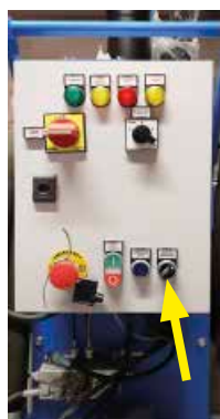
Start/Stop auxiliary pump for particle counter
